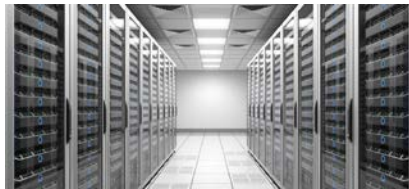
Data Center Management
